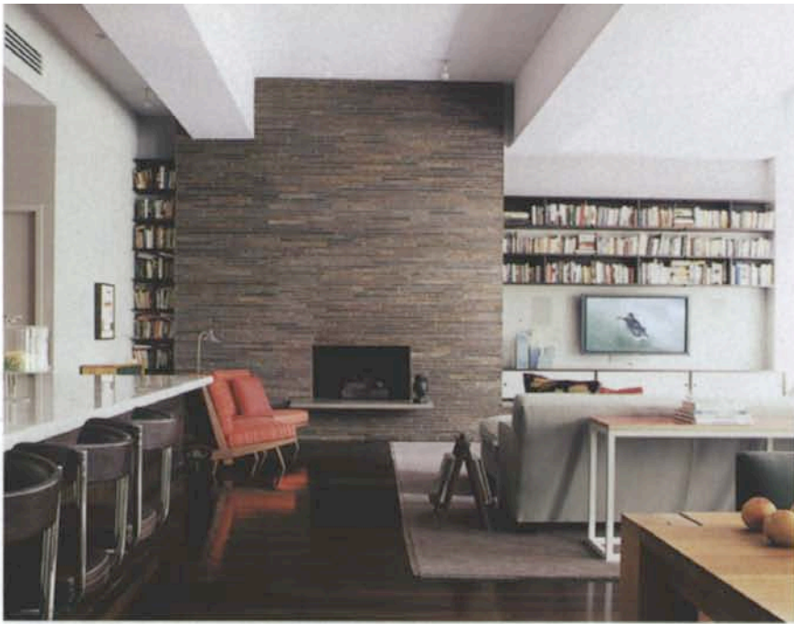
Top: After removing a colonial mantelpiece, the designers modernized the fireplace wall with courses of Kashmir slate floor tile—sawed to 1, 1.5, and 1.75 inches wide—and a cantilevering limestone hearth. Right: The apartment's main seating area features a Dufner Heighes end table and sofas, a custom black-walnut cocktail table, a junk-store lamp, and a hand-knotted Tibetan-wool rug. Bottom: Lulu deKwiatkowski's linen covers the cushions of the living area's vintage George Nakashima chairs.
